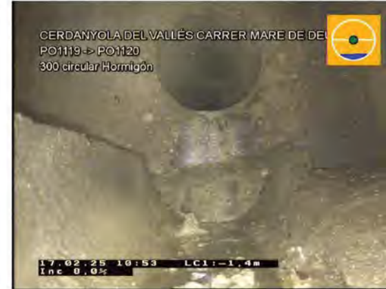
17_02_2025 10_00_01_3f805587-61f4-4b6c-8619-030b4e4eb31a_202502 17_105347_117.jpg, 00:02:44, 34.80m Nudo de final, registro,, PO1119
